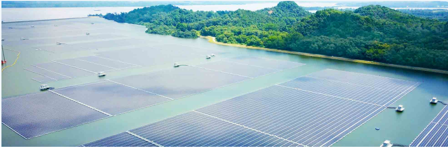
Solar PV system on Tengeh Reservoir, one of the world's largest inland floating solar farms.
